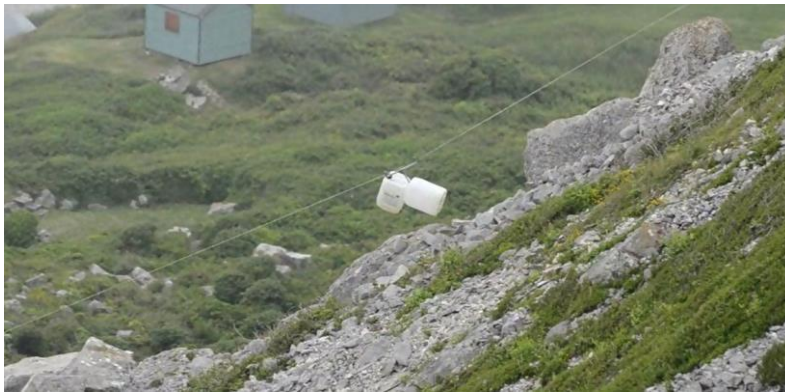
Moving water for chemical treatment by zipline and hose to the most remote areas
